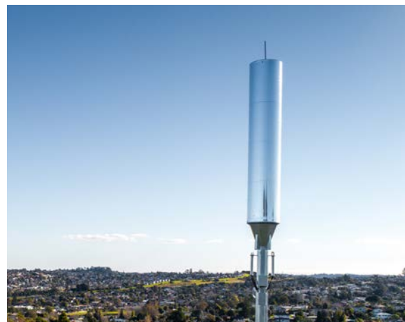
Most new cell towers will be smaller and less obtrusive
