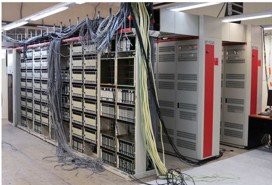
PSTN switches being decommissioned.
